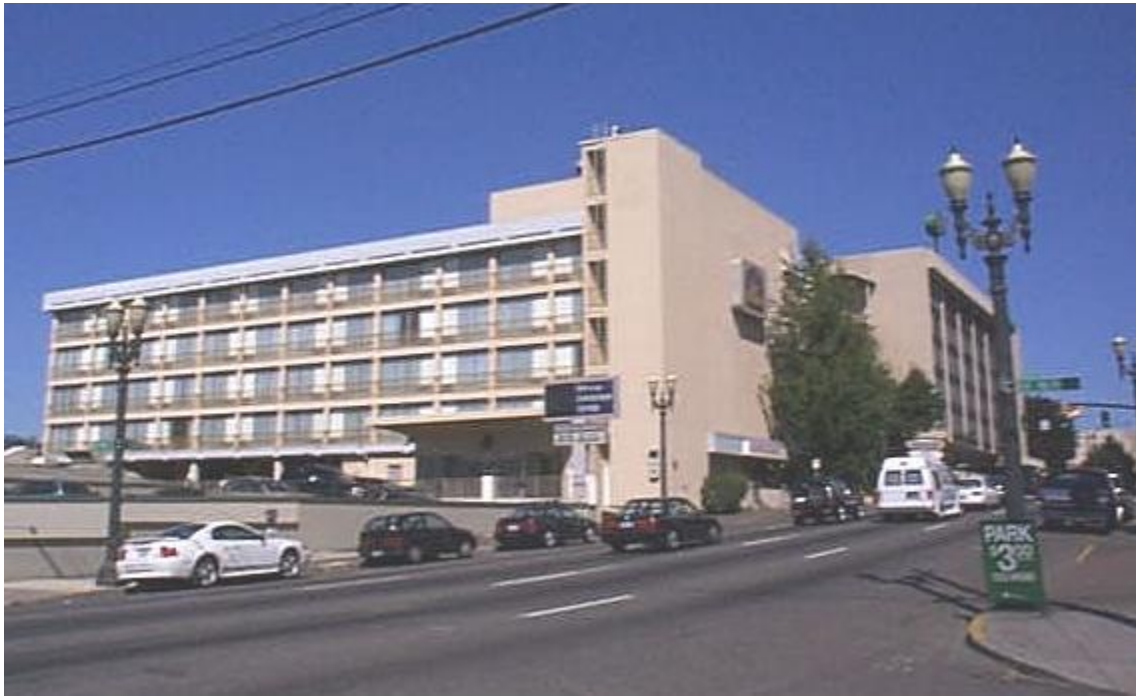
Photo of the Inn at Convention Center looking to the northwest
