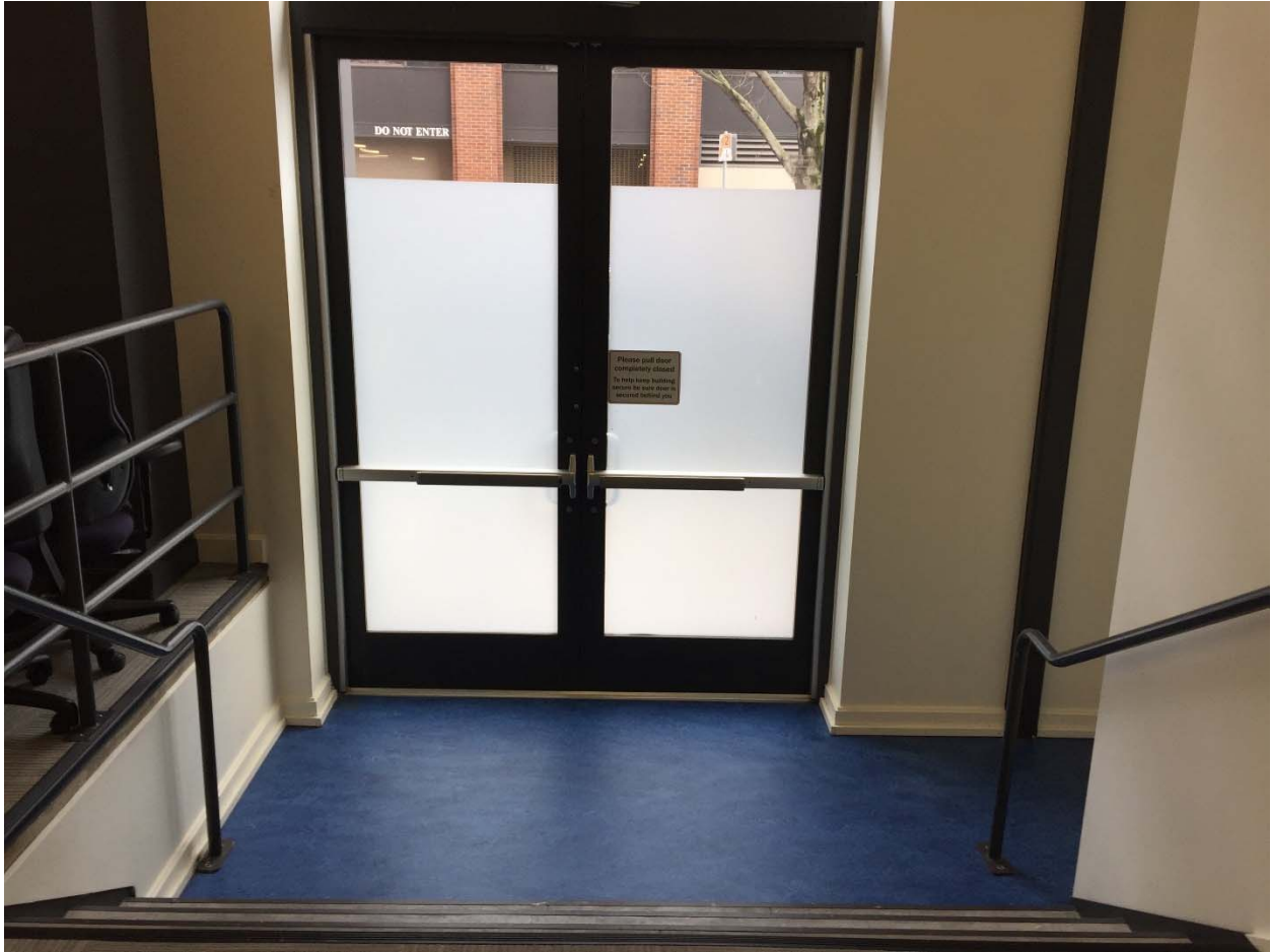
Entryway on the first floor in the Green Room
