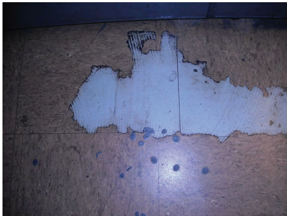
Photo 5. Vehicle maintenance shop office floor with two layers of asbestos-containing floor tile and mastic.
