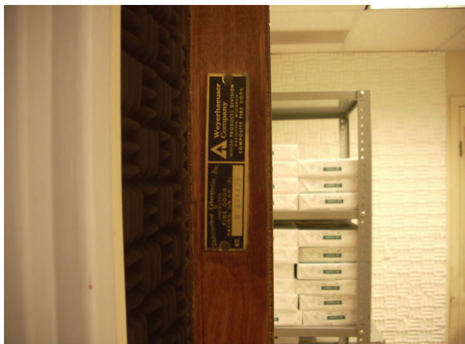
Photo 8. Labeling on a typical asbestos-containing fire.
