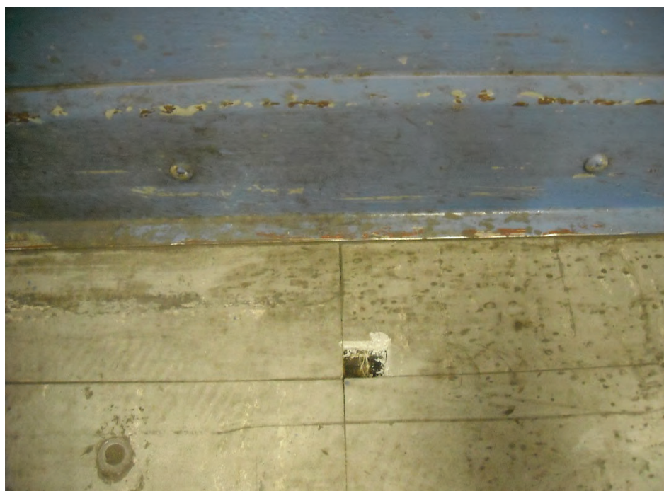
Photo 6. Room 129 asbestos-containing floor tile and mastic. Core sample location.
