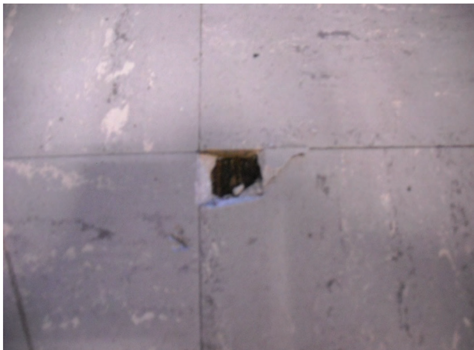
Photo 7. Room 3041 asbestos-containing floor tile and mastic. Core sample location.
