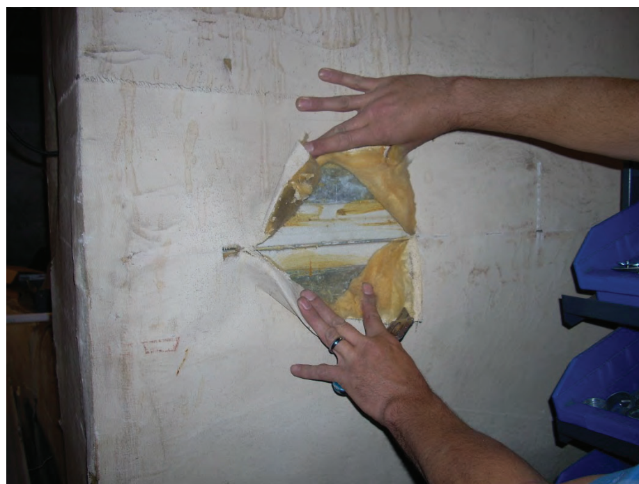
Photo 2. Asbestos-containing duct tape concealed under duct insulation.
