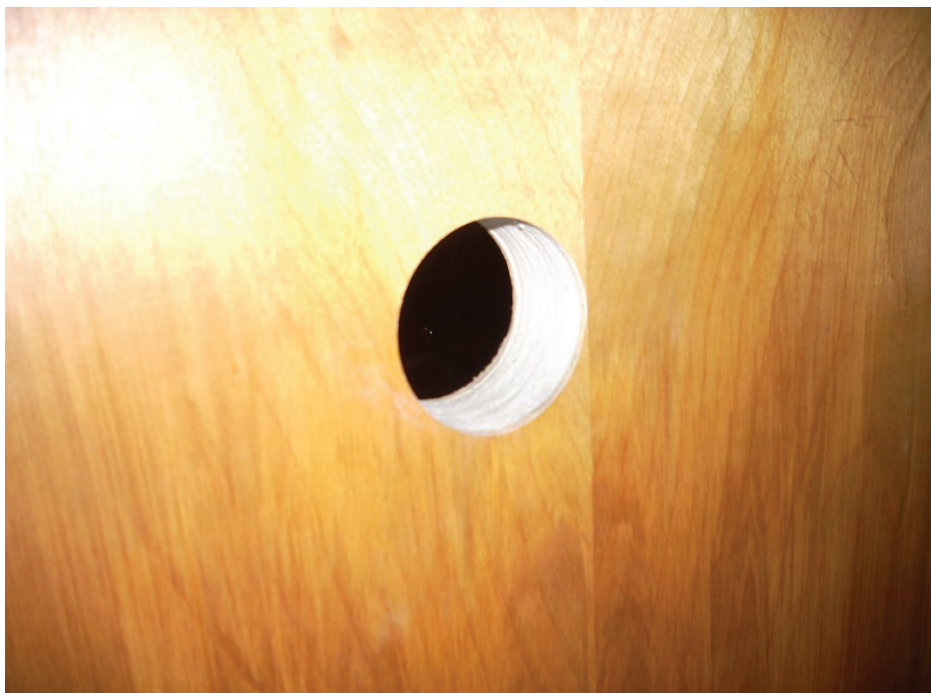
Photo 1. Fire door in tunnel system with exposed asbestos-containing core.
