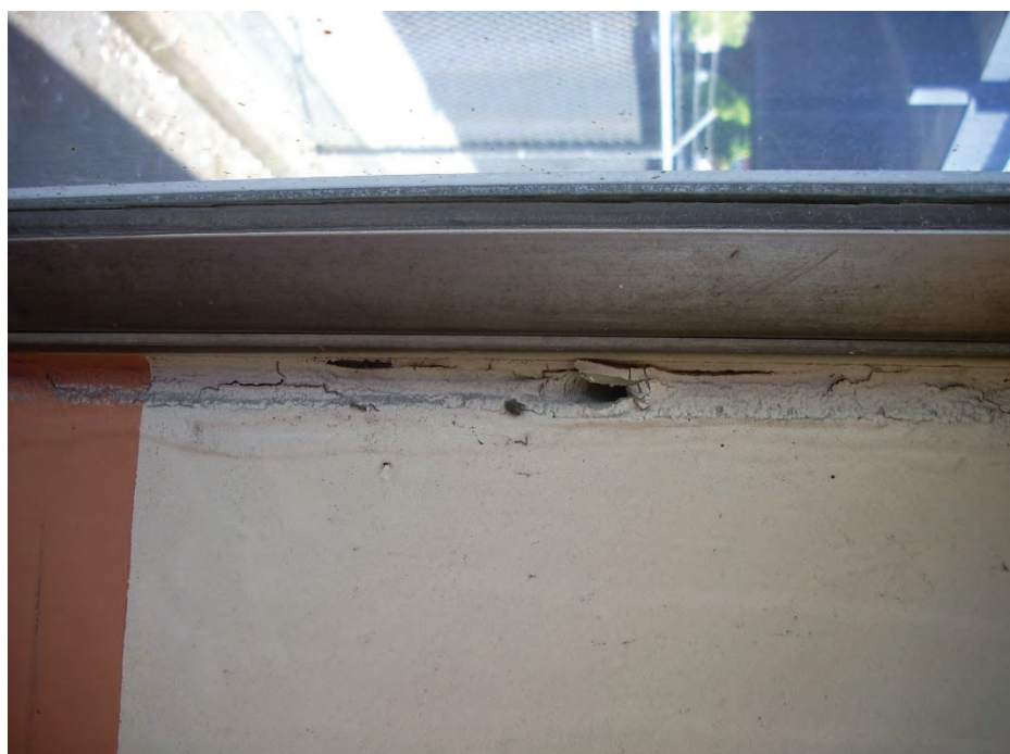
Photo 4. Vehicle maintenance shop window frame with asbestos-containing sealant between the frame and concrete.
