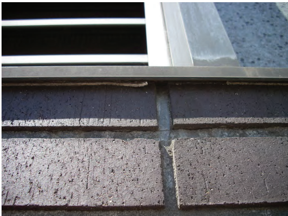
Photo 3. Asbestos-containing sealant between exterior flashing and brick.
