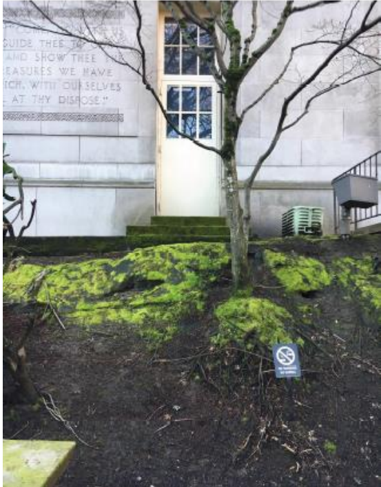
Current emergency exit and landscaping
