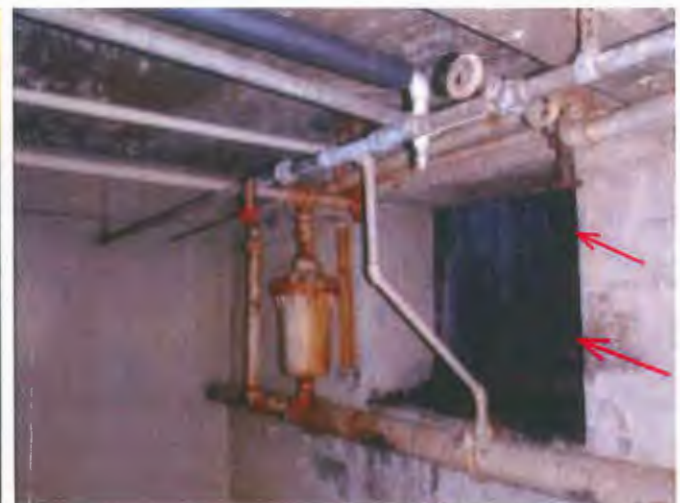
Perhaps originally the northwest basement area had a coal chute?
