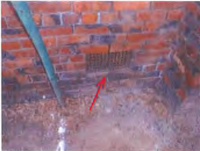
South side abandoned vents for the basement boiler room area.
