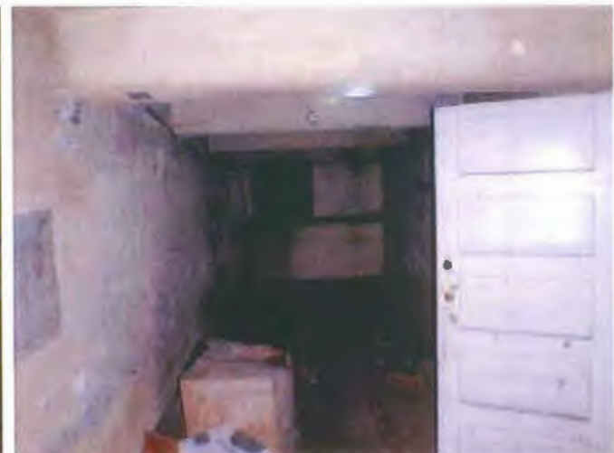
The basement area is built with reinforced concrete.
