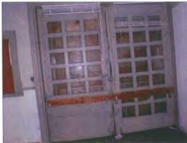
The old fire station front fire truck doors.
