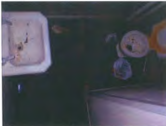
Top floor rest room.
