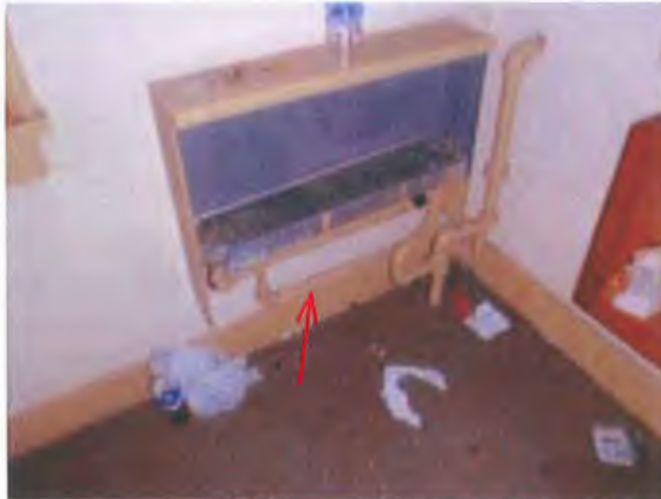
Another more modern hot water heat radiator that's been abandoned.
