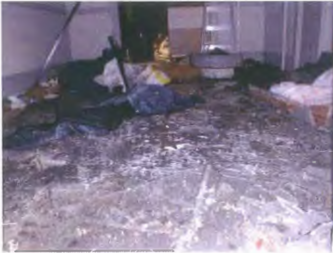
The building needs an amazing amount of clean up and repair.
