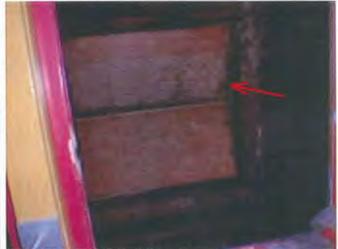
The old original roof skylight has been removed and hole sealed with plywood.
