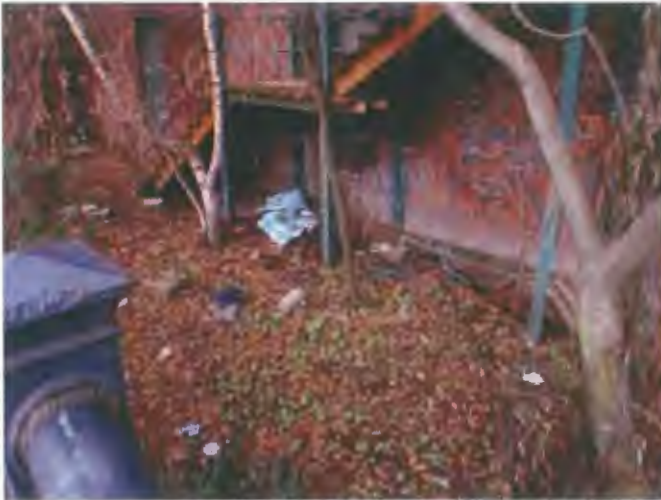
Wider view of the building's south side and stairs to the top floor.
