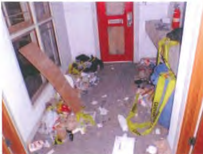
Front entry lobby area.
