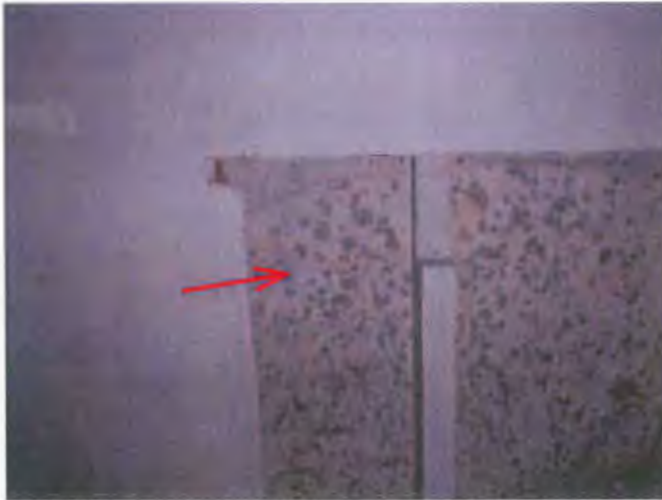
Mold developing all over but much worse on the south side. Roof needs immediate repair.
