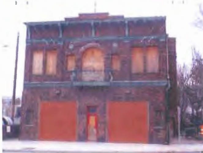
Front Elevation. Building faces west.
