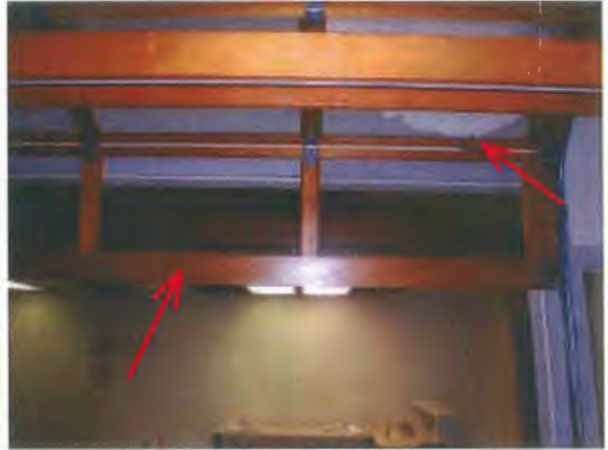
They broke the windows but did not tear down the upstairs "garage" door.
