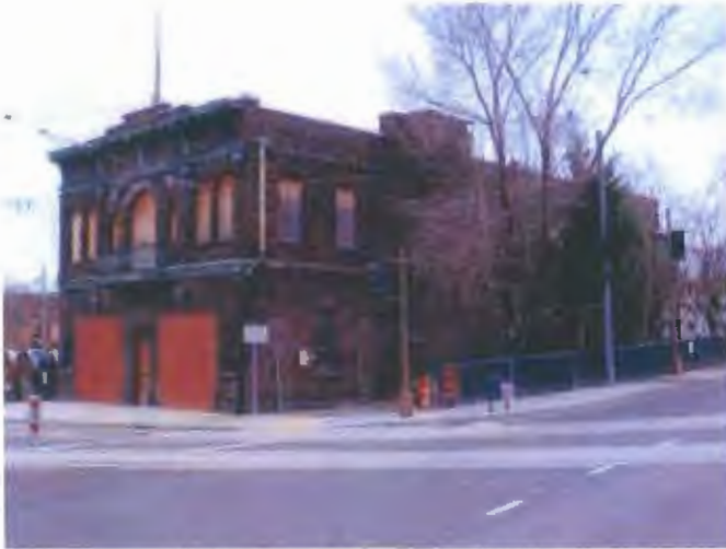
Southwest view. The old building looks pretty good from a distance but needs lots of work.
