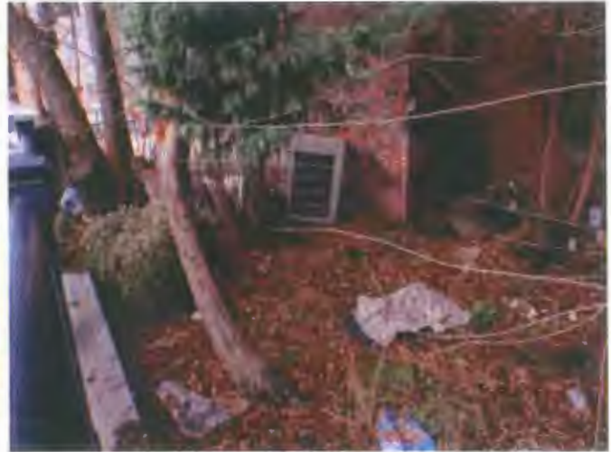
West end of the south side yard and additional mess and damage needing clean-up.
