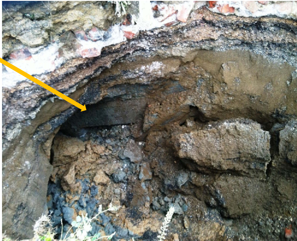
Buried Pile Supported Beam in TP-1
