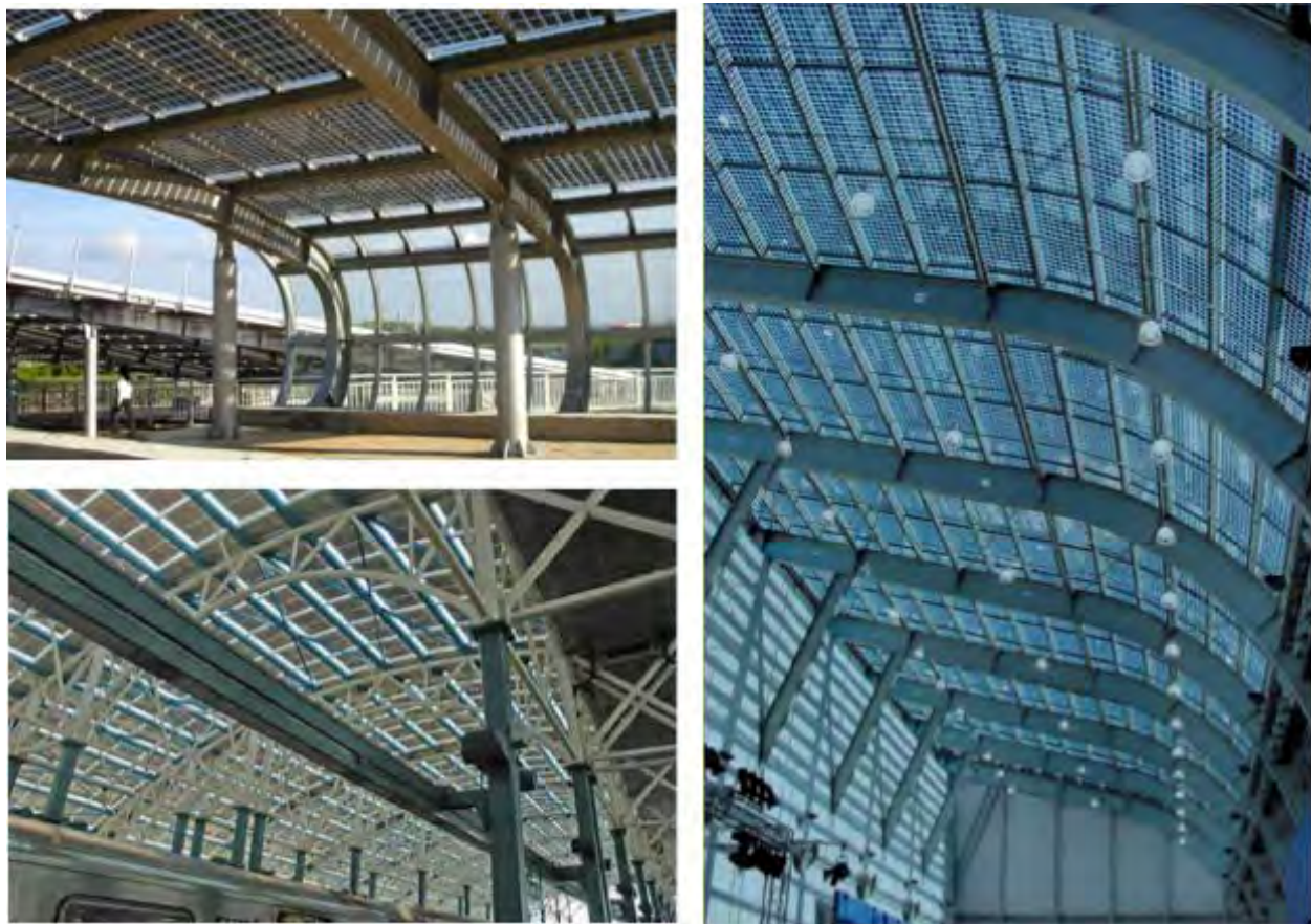
Figure 7.1-2 Examples of Glass Canopies with Embedded Photovoltaic Cells
