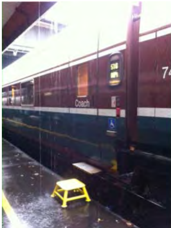
Figure 7.1-6 Insufficient Passenger Weather Protection of Existing Canopies
