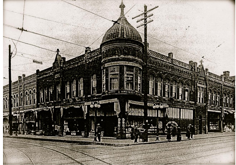
Hill Block Building
