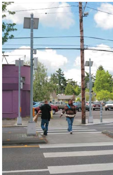
An RRFB on SE Foster just east of SE 80th Avenue. Source: PBOT
