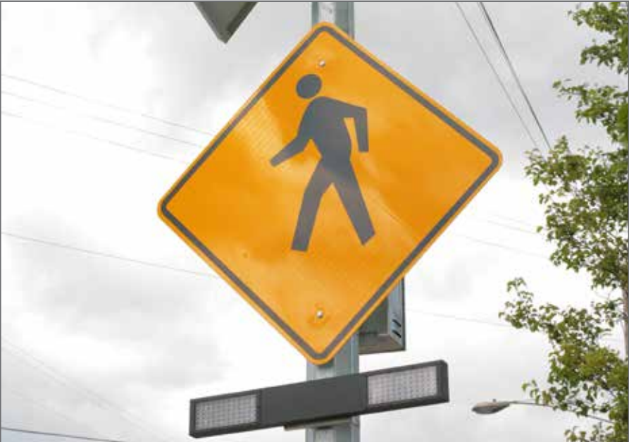
Close up of the rectangular rapid flashing beacon head and signage.
