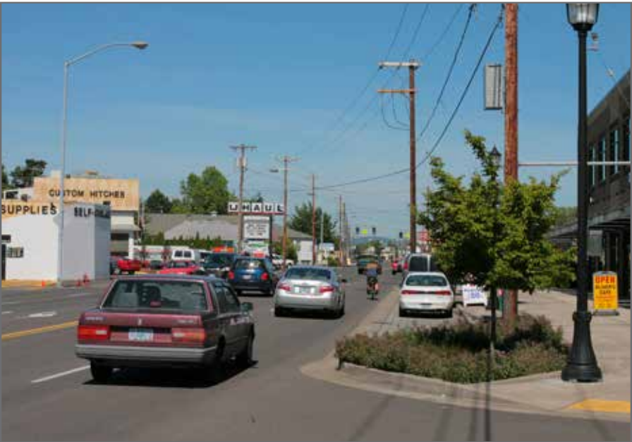
A curb extension on Foster Road at SE 92nd Avenue reduces crossing distances and expands the amount of programmable space for street furniture, lighting, and plantings.
