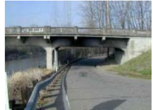
Schmeer Rd undercrossing of Denver Ave.
