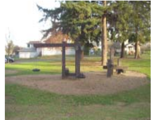
Trenton Park - old wooden play structure is in need of replacement.
