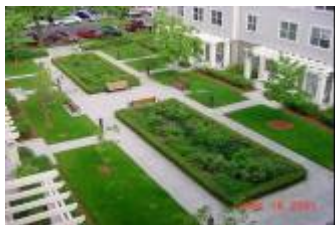
Courtyard infiltration basin at Buckman Heights Apts.
