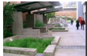
Stormwater planters to underground rainwater harvesting system
