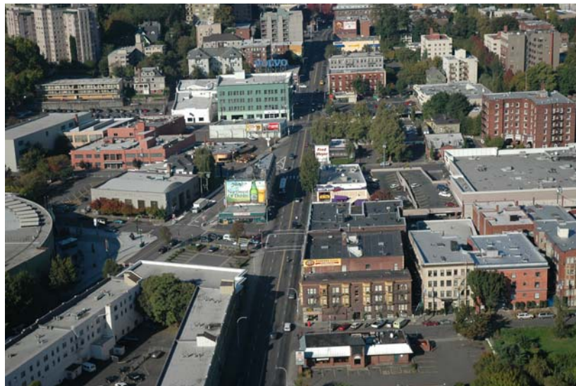
The above photograph shows Burnside west from SW 19th. This stretch of Burnside would have four 10-foot travel lanes, new 10-foot sidewalks, ornamental street lights and street trees on both sides of Burnside.
