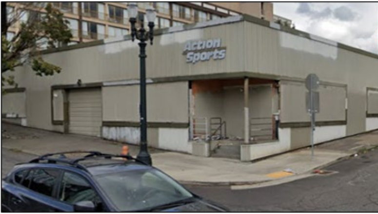
Current Project Site
