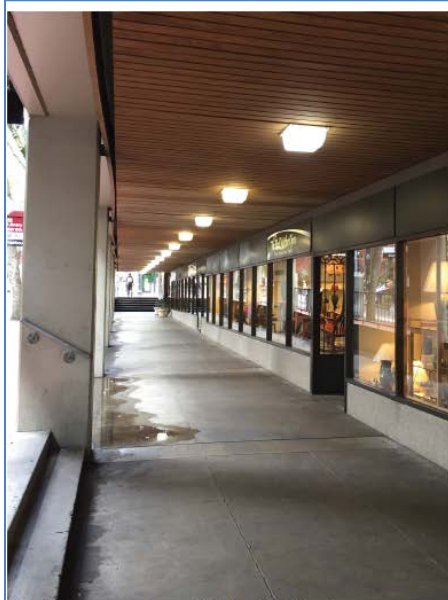
Existing arcade along SW Yamhill Street.
