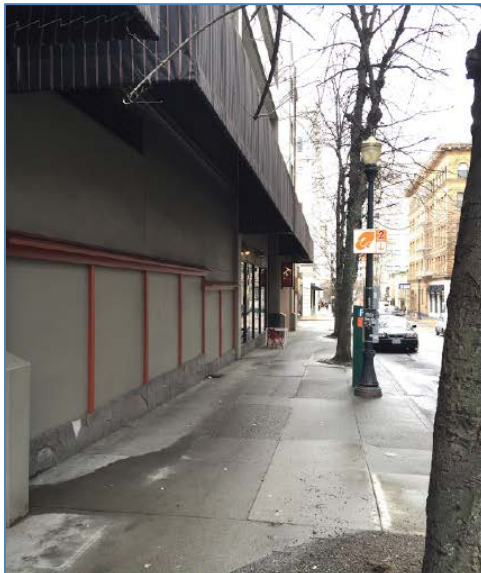
Existing facade along SW Ninth Avenue.
