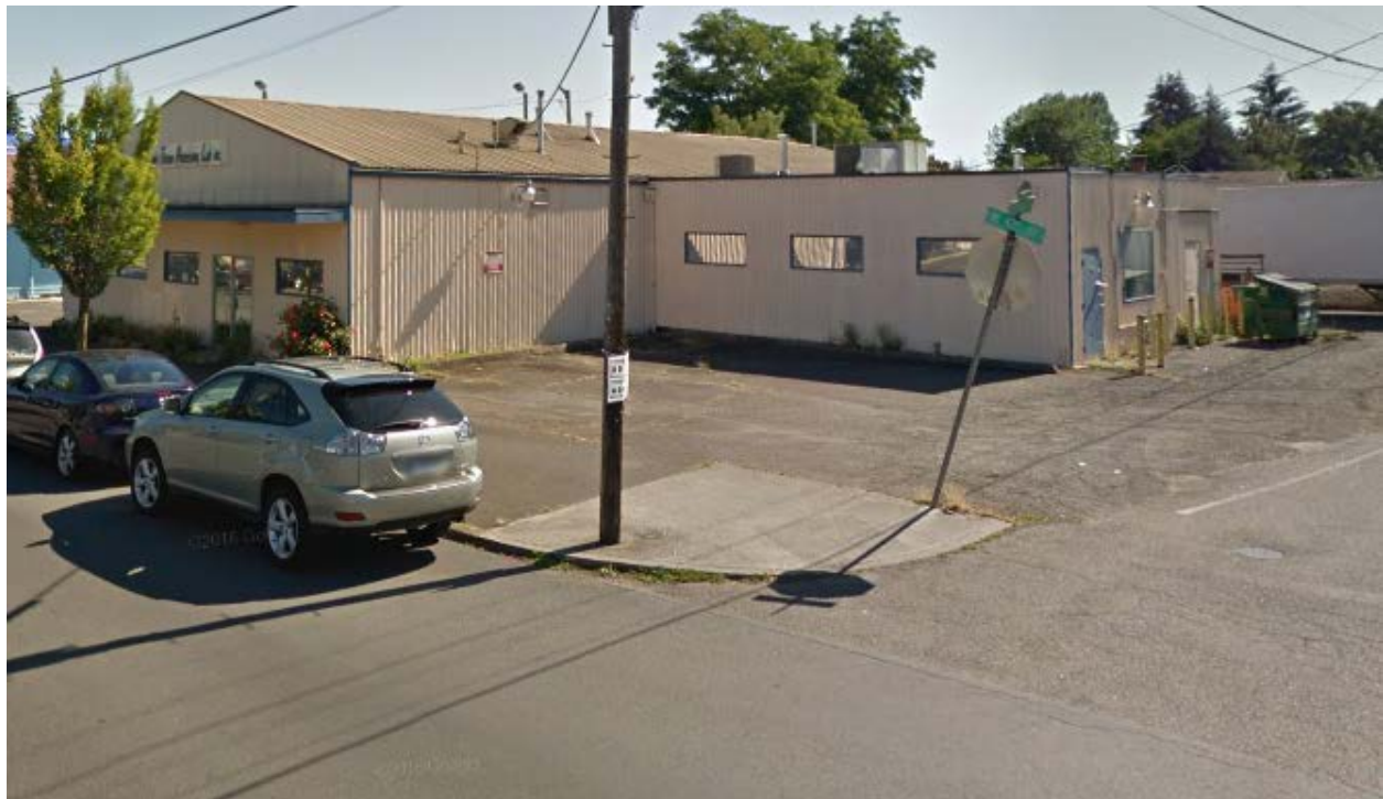
View from NE 42 nd and Alberta, Looking Northeast
