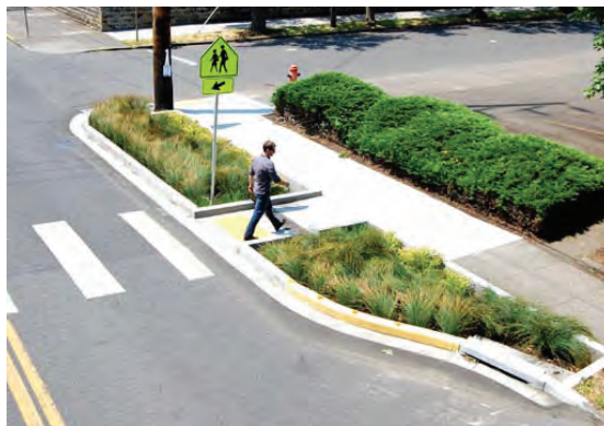
Stormwater curb extensions
