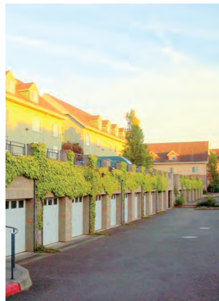
Two-tiered parking deck at Russellville Commons.
