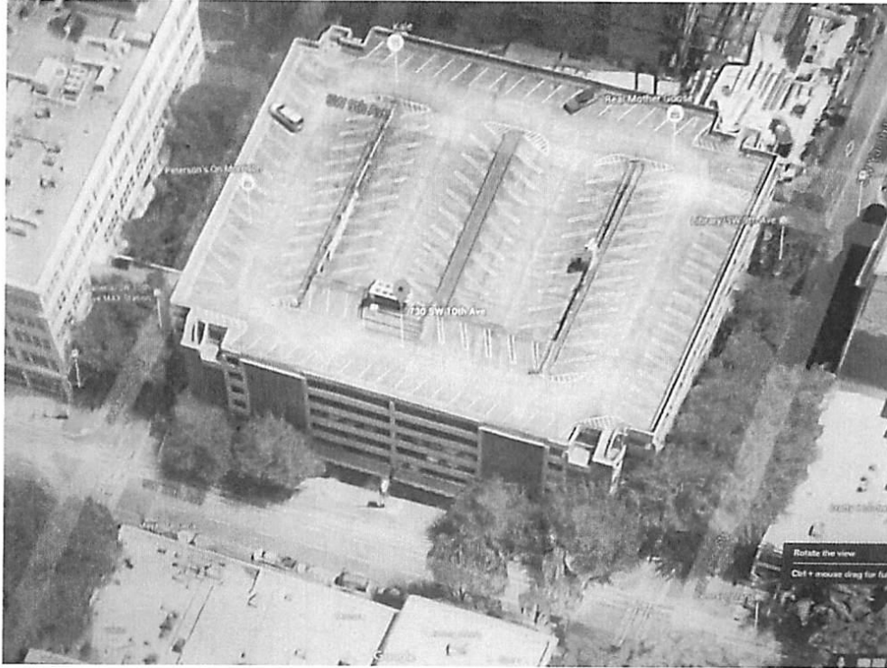
Figure 1, Overview of the Garage Building (Source: Google)
