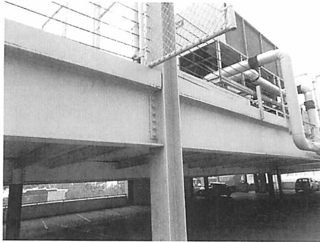
Figure 2, Steel framing in the upper floors
