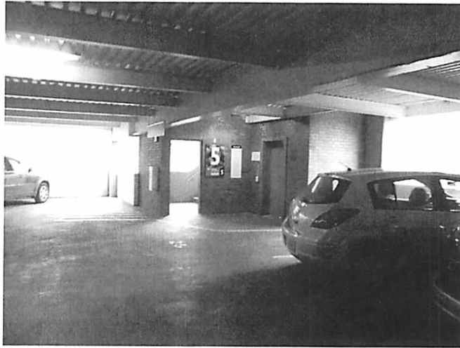
Figure 8, Framing system in the 5 th floor
