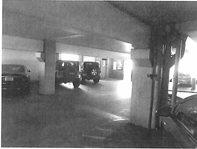
Figure 10, Concrete framing system in the 3 rd floor
