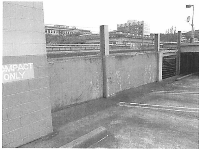
Figure 7, Shear walls in the E-W direction
