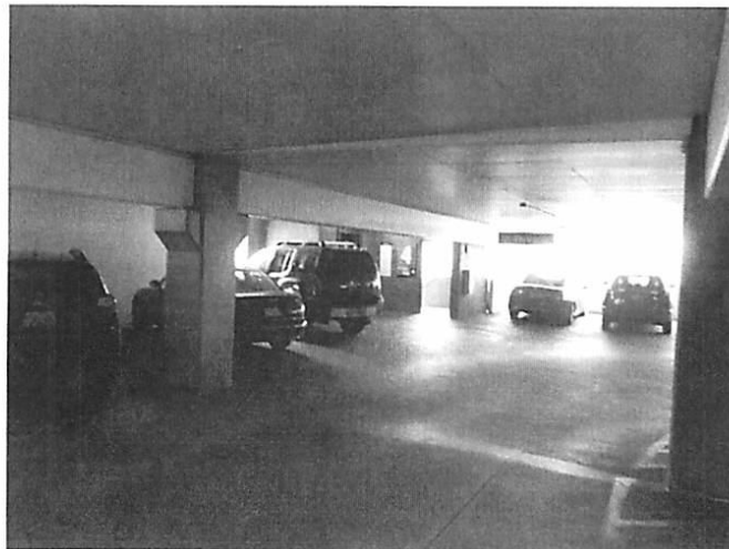
Figure 9, Concrete framing system in the 4 th floor
