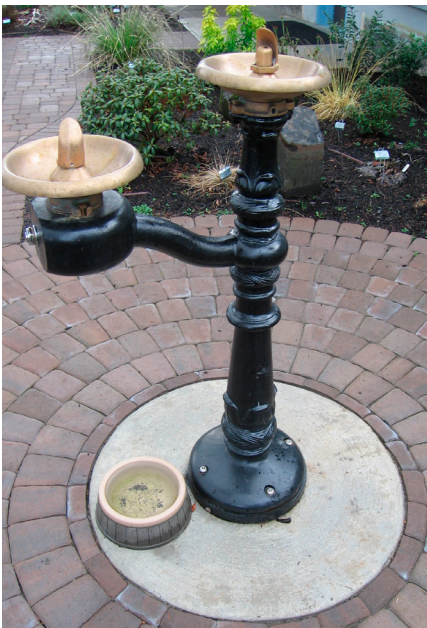
Portland Water Bureau decorative drinking fountain, shown here during installation in the Hazelwood Hydro Park
