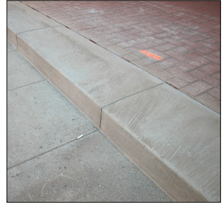
Recommended: 12-inch Concrete Curb (Portland Mall)
