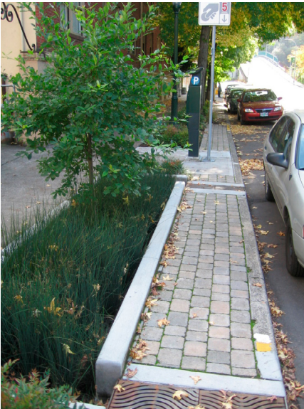
Existing stormwater planter at SW 12th and Montgomery
