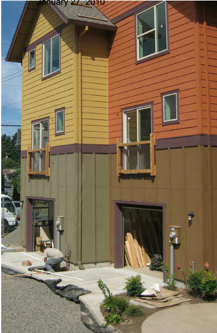
Pardee Commons, a PDC housing project, under construction.
