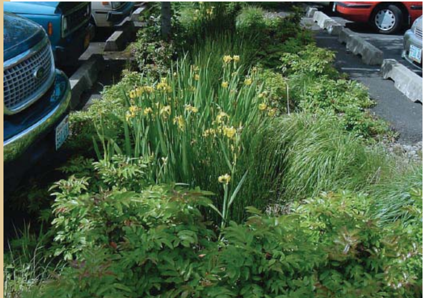
Bioswales collect and filter hardscape runoff.
