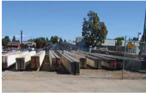
Two dozen massive 40-foot long, old growth Douglas Fir beams salvaged by Konell Construction from a warehouse on Martin Luther King, Jr. Blvd, await transfer to be re-milled for reuse.
