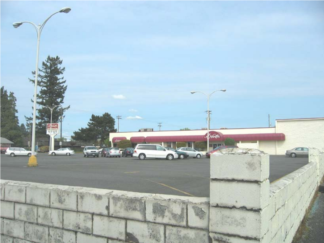
10520 NE Halsey Street (Parcel 3)
