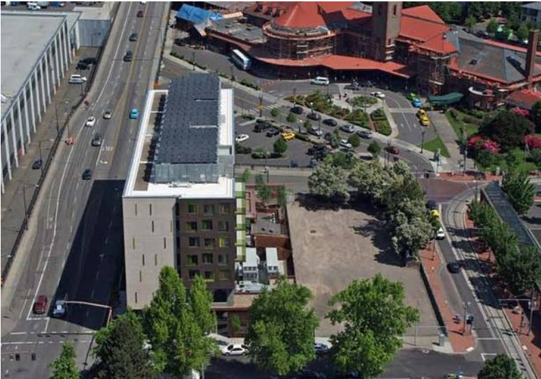
Site is on the vacant block edge in the photo below
