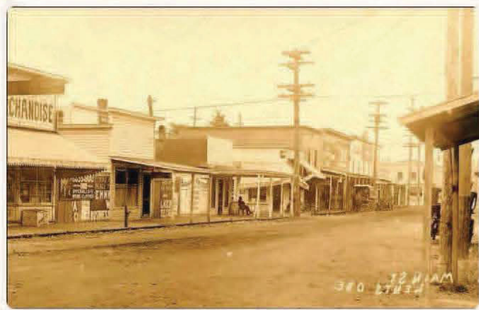
Photo: View of Main Street or 92nd Avenue looking north from Woodstock
