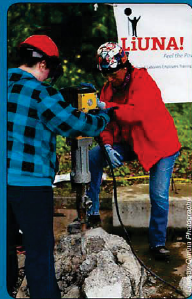
A high school girl learns to operate a jackhammer from Aida Aranda, Apprentice Coordinator for the Oregon & Southern Idaho Laborers-Employers Training Trust
