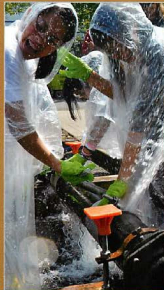
Middle school girls have a blast as they try to stop the break and shut off the flow of water in the Portland Water Bureau's "Fix a Water Main" workshop.
